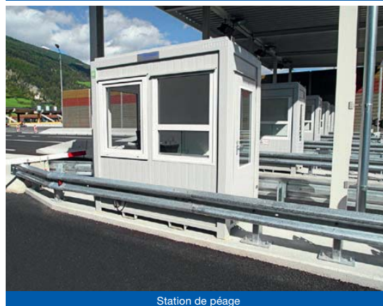
Station de péage
